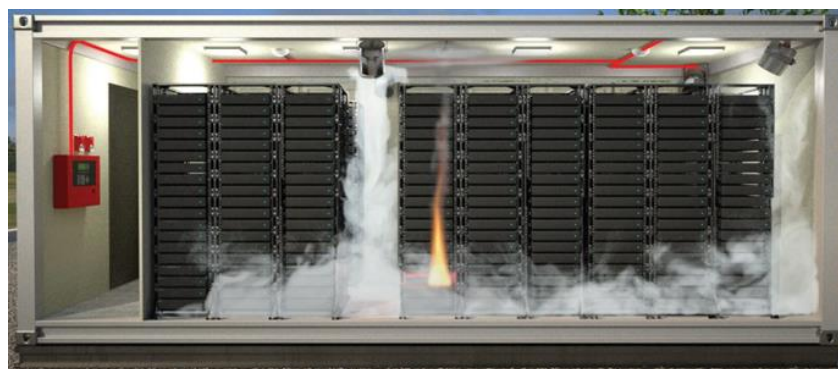
Figure 24: Example Showing Discharge of Suppression Agent
